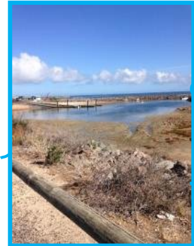
Port Hughes Jetty
